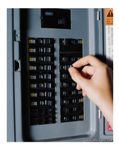
operating an appliance with too high a voltage or wattage requirement for the circuit. The sudden starting of an electric motor can also trip a breaker. If a breaker trips repeatedly check for any of the above causes.
